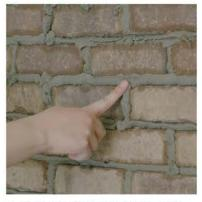
5. Start at the top of your wall. Fill in sections of about 4 square feet at a time. Give each section about 15 minutes to dry. You can do about 4 sections one after the other before going back with your brick jointer. When the grout is dry enough to touch without sticking to your finger, it is ready to start tooling. It should still be soft enough to compress a little.
