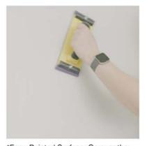
\*For a Painted Surface: Go over the wall with some 80 grit sandpaper. Use a small circle motion and go over the entire surface of the wall. You don't need to push hard, the goal is simply to rough up the surface so that your adhesive improve bond.
