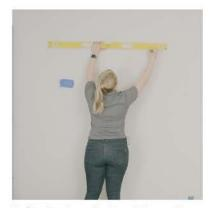
Starting from the top of the wall, measure down at 21" increments. Mark horizontal lines on the wall using a level. Apply adhesive and thin brick section by section.
