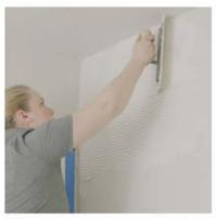
Use a notched trowel to apply the adhesive. Smear on the adhesive generously with the flat side first and then use the notched side to scrape off excess.
