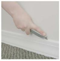
2. Remove any baseboards and trim that are less than ½" thick. To remove a baseboard, start by scoring the caulk with a box cutter or other sharp knife.
