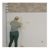
For the edges, you can remove bricks from a sheet and cut them to size with a hand-held tile saw.
