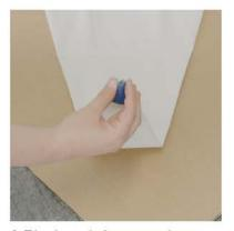
2. Trim the end of your grout bag so that the opening is about ½" wide. Then fill your grout bag by folding down the top edge of the bag and then step on the tip of the bag. Use a trowel to fill the bag about half-way.
