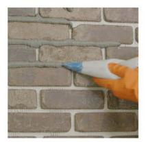
4. Hold the grout bag with one hand in the middle and one hand at the end where it is twisted. Put the tip of the bag in the space between the bricks at a 45 degree angle. Twist the end of the bag and squeeze as you move the tip along the gap. The grout should over fill the gap just a little so that you have enough to tool later. This process takes some practice. \*Do not try to wipe off excess while the grout is wet.\*
