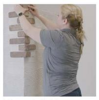
If your project includes corners, install your corner pieces first starting at the top of the wall using the following steps. After the corner sheets are installed use these same steps again to install flat sheets.
