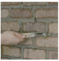
6. Use the heal edge of your jointer to push the mortar into the gap and away from you. The excess mortar should fall away and not stick to the brick face. If the mortar is sticking, it is still too wet and needs to set for a few more minutes. You should get clean edges with a slight indent in the grout.
